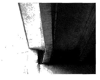
Work to carry out essential structural repairs to Primrose Hill bridge following a bridge strike that resulted in significant deformation of several primary beams.
