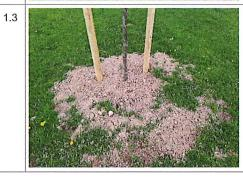
Gele Park – bark mulching still requires completing. Irrigation pipe pulled out of tree pit shown and quite a few caps missing. Irrigation pipes need cutting back so less vulnerable.
